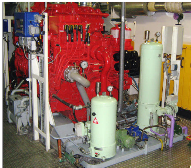
MTU diesel engine type 12 V 4000 M53 with installed CJC® Fine Filter Unit 27/54 (le) for lube oil filtration and CJC® Filter Separator 27/108 (ri) for diesel filtration.
