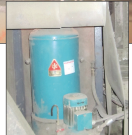
CJC® Fine Filter Unit 27/54 installed at Trunnion FIXED and FLOATING bearings
