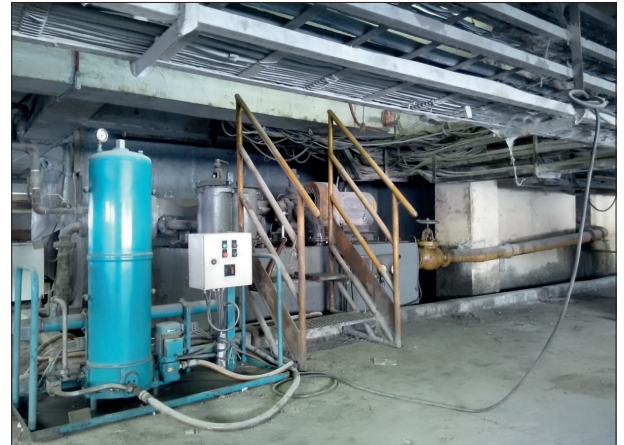
Republic Cement Iligan, Inc. - Gearbox of finish grinding mill no. 1 with installed CJC™ Fine Filter unit 27/108.
