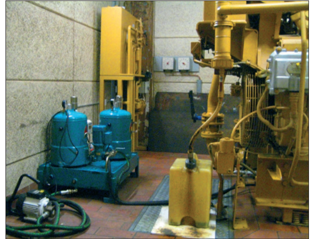
E.ON Danmark A/S, Caterpillar Gas Engine and the CJC® Lube Oil Filter 27/27-27/27
