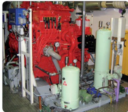
CJC™ Fine Filter unit (left) for lube oil filtration and CJC™ Filter Separator (right) for diesel oil filtration installed at the MTU engine
