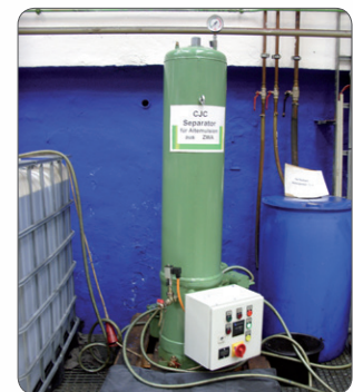
CJC™ Filter Separator installed at intermediate bulk container
